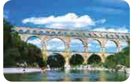
Roman aqueduct (France)
