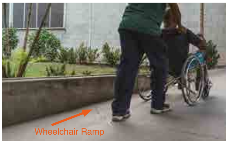
A ramp makes it easier to push the wheelchair up.
